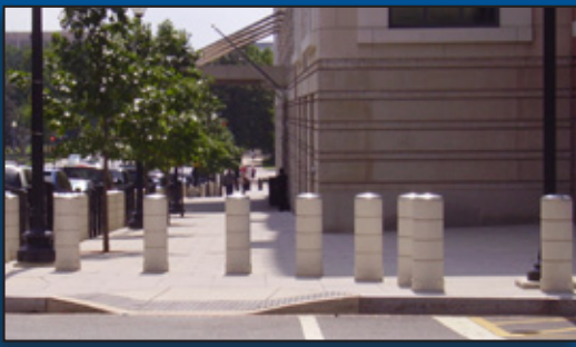
GFRC Bollards, U.S. Capitol
