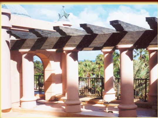
Rooftop pergola or belvedere with FRP columns and fiberglass texture wood beams.
