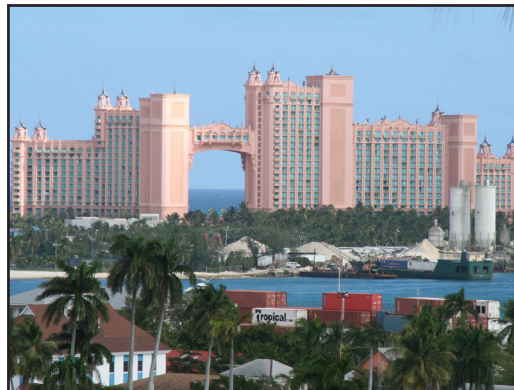
Atlantis Resort • GRC Panels
