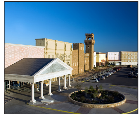
Winstar World Casino • GRC Wall Panel System
