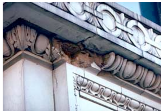
Material spalling is the result of excessive expansion of the porous tile body caused by water and freezing temperatures. This is a serious condition, often difficult to repair. Photo: NPS files.
