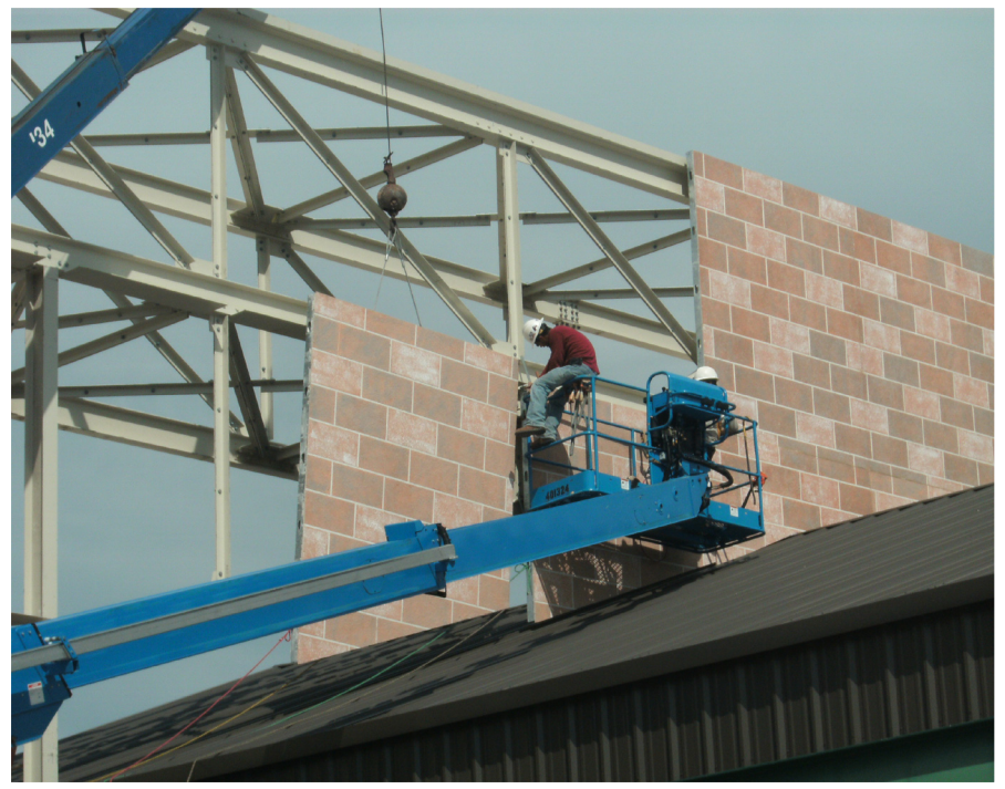
Panels being installed
