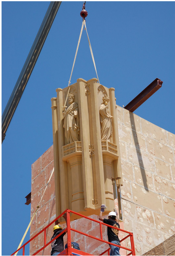
Installation of GFRC panel
