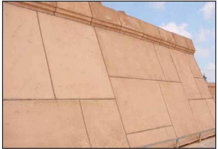
Ashlar panels, Stromberg GFRS (glass fiber reinforced stone) a type of architectural fiberglass, Atlantis, Bahamas.
