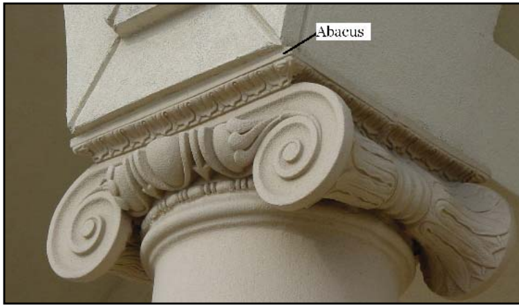
Abacus of a Roman Ionic Column Capital cast in GFRC
