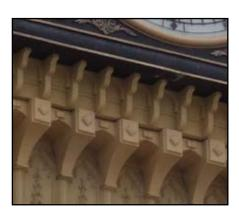
fiberglass) brackets may be molded into the cornice, or applied as separate pieces.
