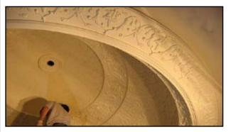
Ornamented ceiling dome being installed (GFRG)
