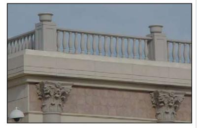
Balustrade as parapet wall • Architectural Fiberglass (GFRP)
