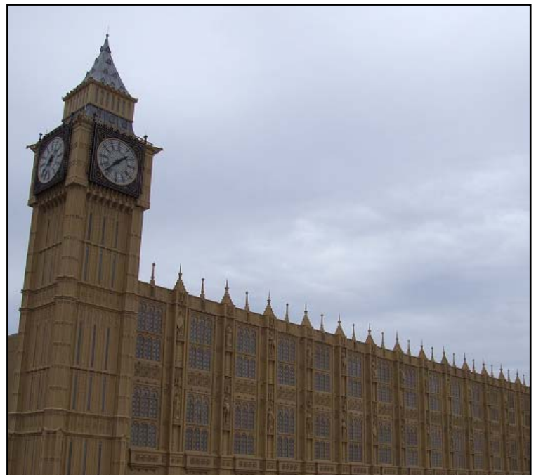
Gothic revival style facade in architectural fiberglass
