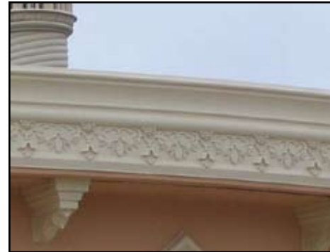
Corbels supporting a cornice
