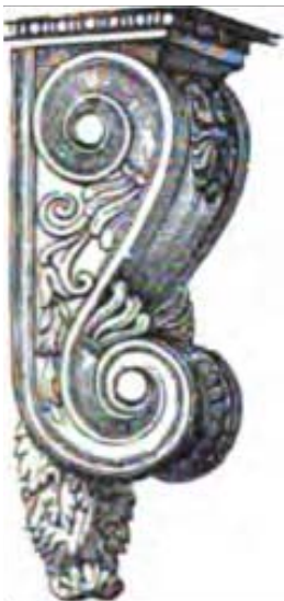
Ancon (a console or scroll shaped bracket)
