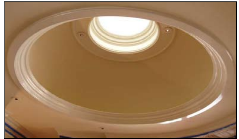
Dome in GFRG
