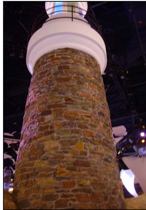
Fieldstone panel for "lighthouse" cast in GFRC (glass fiber reinforced gypsum) for interior use. Fieldstone panels could also be cast in architectural fiberglass or GFRC for exterior use.
