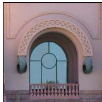
Arch cast in Stromberg architectural fiberglass
