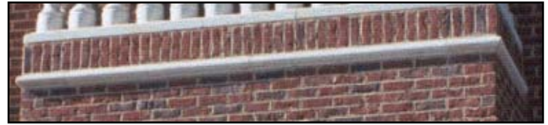
Band or band molding. The horizontal molding, projecting from the surface that wraps around a building. Also known as a belt course or watertable.
