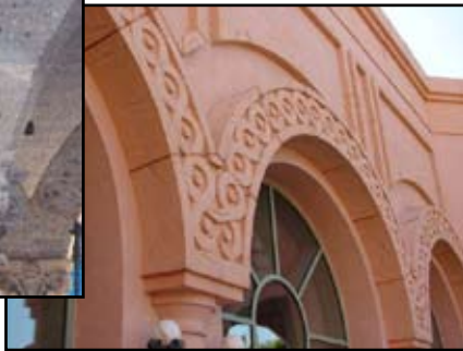
Carved voussoirs or arch stones. Cast by Stromberg in a custom color and texture architectural fiberglass.
