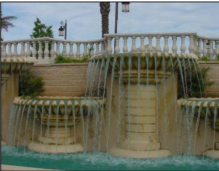
Balustrade at fountain • Style G29 baluster and style W10 baluster railing • Cast stone
