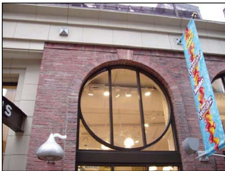
Architectural fiberglass brick panels, Hershey's Times Square, New York
