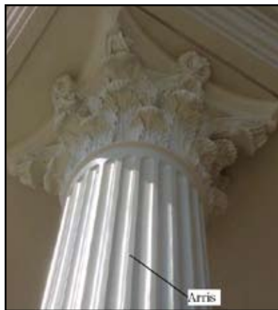
Arris on an architectural fiberglass (GFRP) Corinthian column
