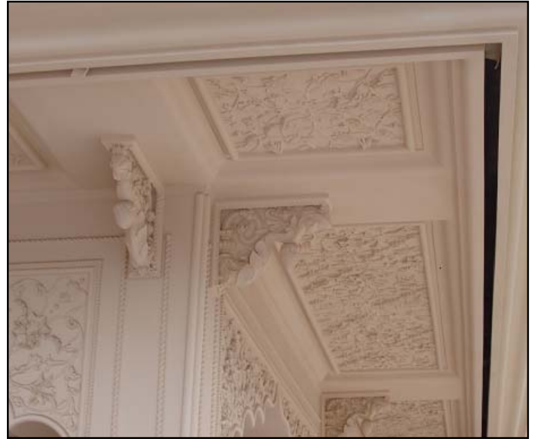
Highly ornamented eaves
