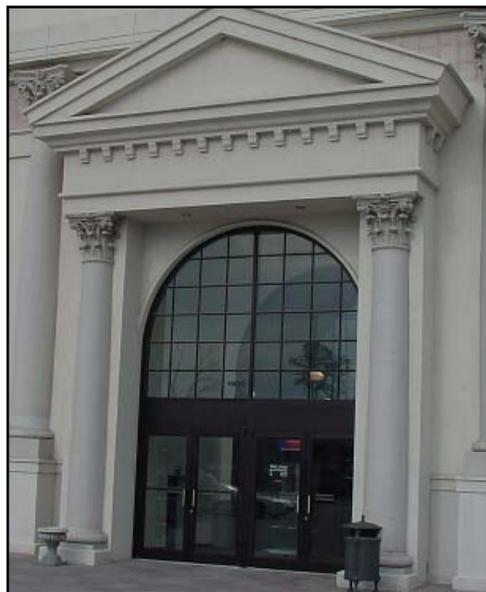
*Corinthian pilasters in GFRC (The Stromberg stone faced architectural fiberglass)*
