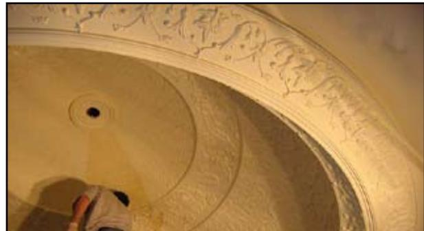
*Ornamented ceiling dome being installed (GFRC)*
