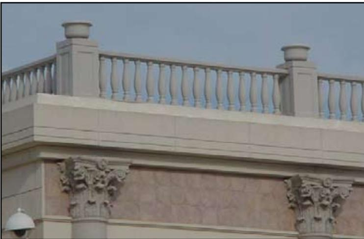
Balustrade as parapet wall • Architectural Fiberglass (GFRP)
