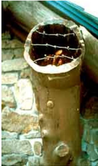
The core of a deteriorated wood outrigger was first drilled out. Photos (left and right): Courtesy, Harrison Goodall.
