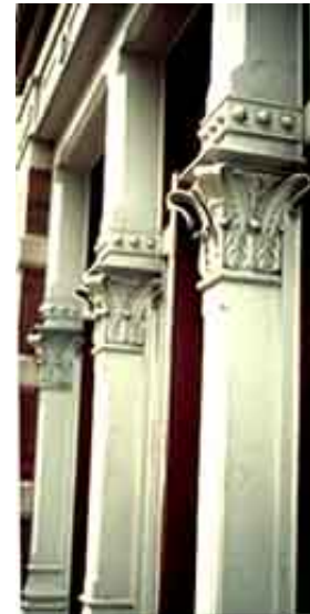
Cast aluminum has been used as a replacement material for cast iron. Photo: NPS files.
