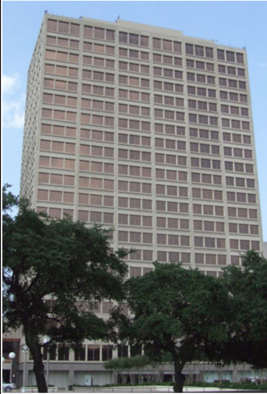
Galleria Tower II GFR C
