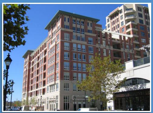
in 8' long sections of GFRC with a cast in limestone finish and an integral metal stud frame. Stromberg's affiliated installation company also provided the installation for this project.
