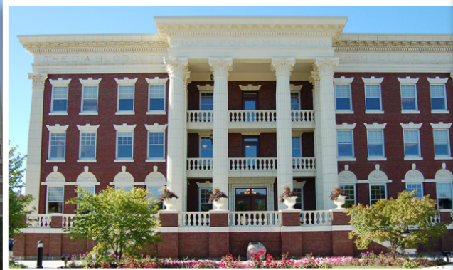
Blodgett Building, Grand Rapids Michigan GFRC and TerraGlas re-clad and replacement of missing terra cotta facade, cornice and columns.
