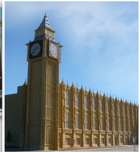
Winstar World Casino Re-cladding of existing casino
