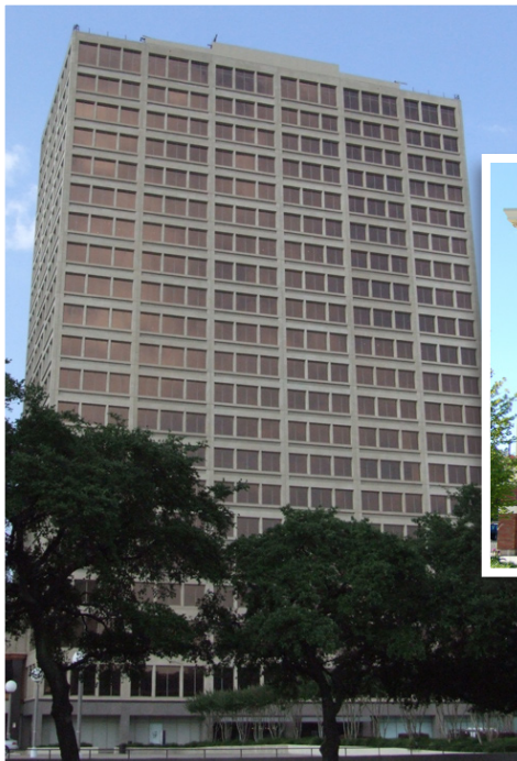
Blodgett Building, Grand Rapids Michigan GFRC and TerraGlas re-clad and replacement of missing terra cotta facade, cornice and columns.
